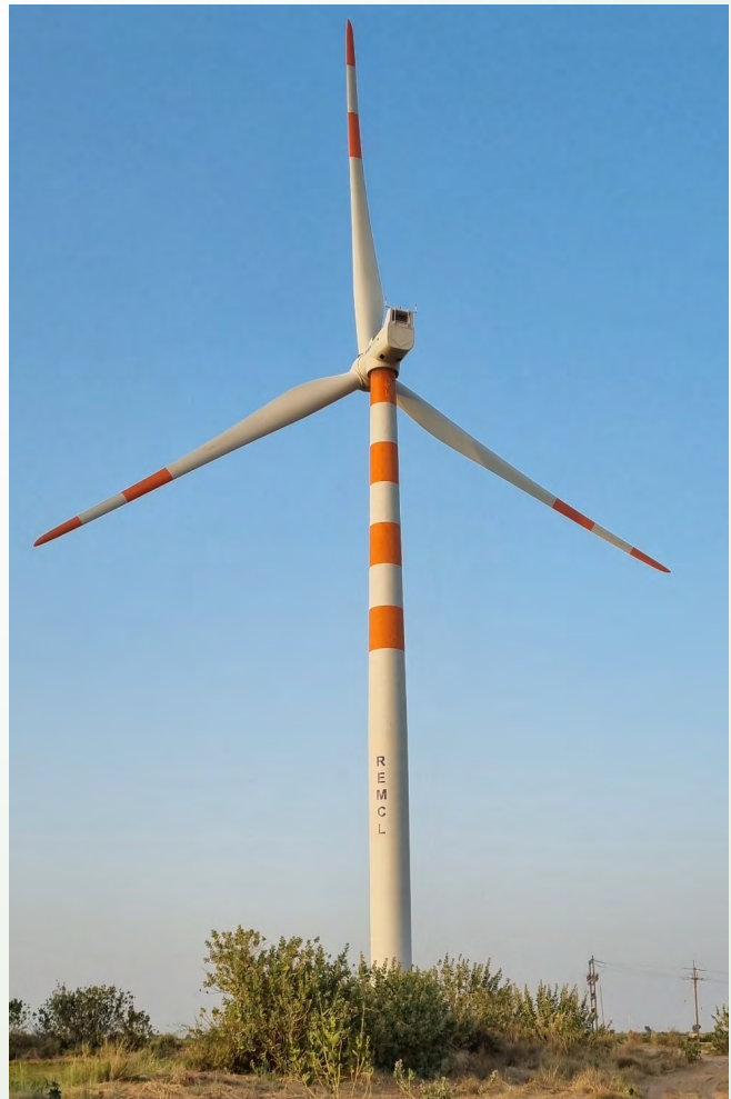
Wind power plant at Jaisalmer, Rajasthan
